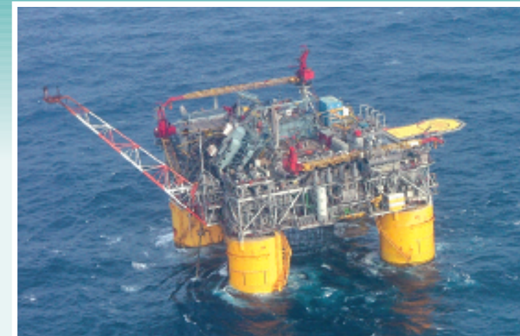
After Hurricane Katrina made landfall, a fixed-wing aircraft flew out of Houston over the Gulf of Mexico to assess damage. The Mars TLP (shown) suffered a toppled drilling derrick.
